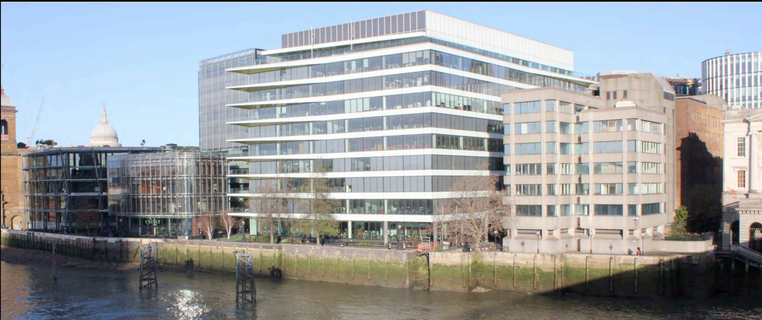
Swan Lane Pier
